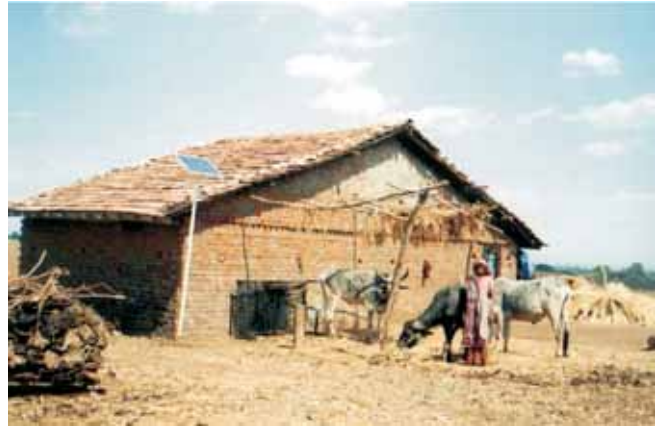
Figure 6 Home light system in an isolated house
